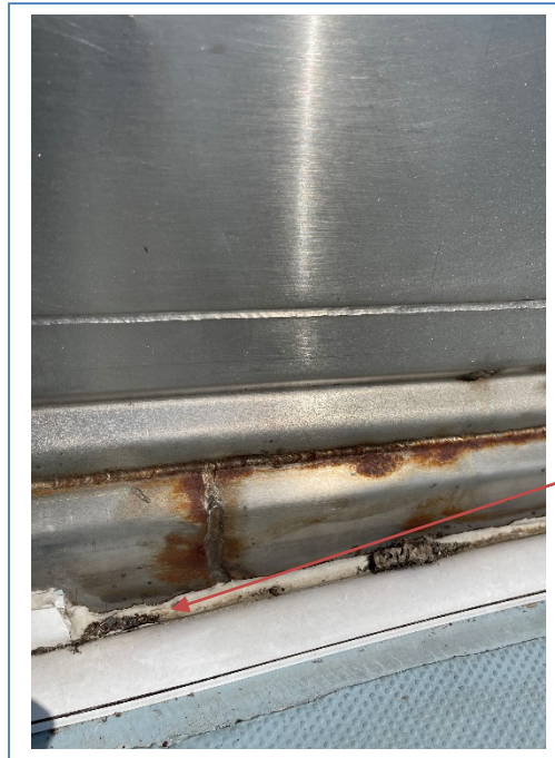
DETERIORATED CAULK JOINT
