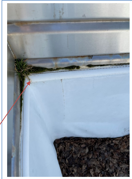
DETERIORATED CAULK JINT
