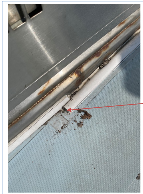
COMPRESSION STRIP INSTALLED INCORRECTLY.
