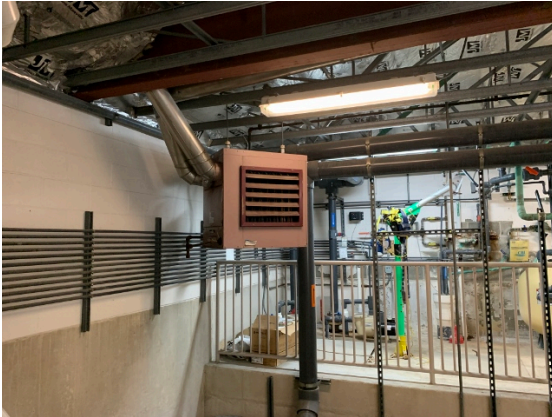
Gas-fired unit heater
