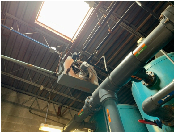
Hot water unit heater
