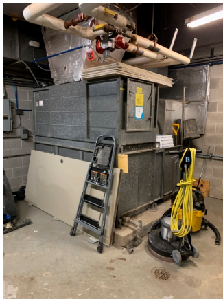
Air handler in Boiler Room
