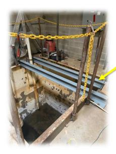
New I-beams installed to mount new pump on.
