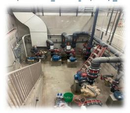
Pumps were not braced properly in the past but are now situated on concrete bases to eliminate the pumps moving in any fashion.
