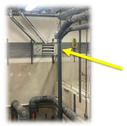
Not only was the overhead heater replaced but it was re-hung to provide better access for routine maintenance in the future. The old unit required scaffolding to service and/or repair while the new unit can be accessed from the existing concrete walkway.
