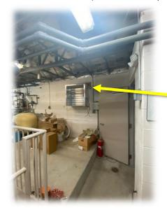
New ventilation in roof and side wall will allow us to sweep air out of pump room and replace with fresh air to slow down the corrosion of all metal fittings throughout the pump room.
